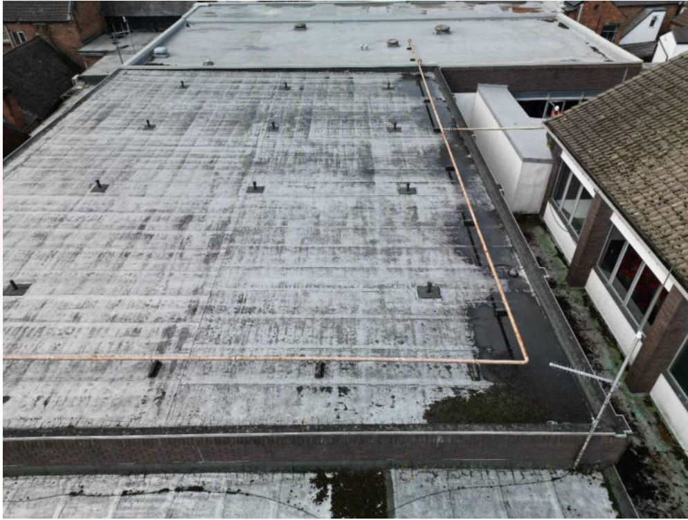
Photograph 24 – Roof over Theatre Hall 2024 for comparison
