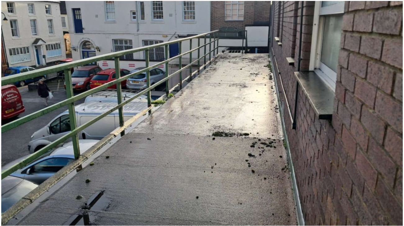
Photograph 6 – Top side of rear walkway
