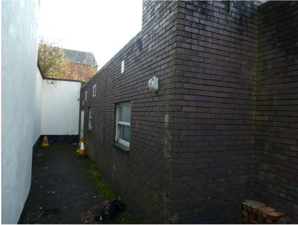
Photograph 8 – Right side elevation of Civic Centre
