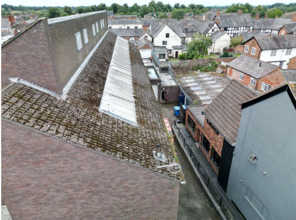
Photograph 28 – Roof over left hand side Market Hall 2024 for comparison
