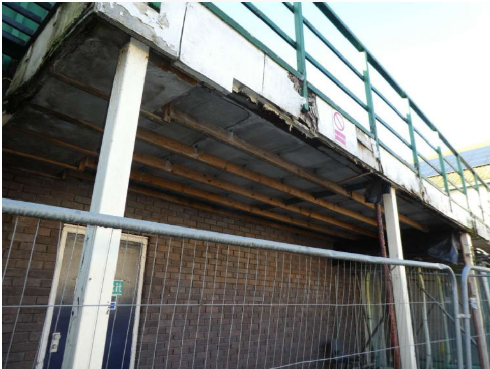
Photograph 5 – Steelwork arrangement to canopy
