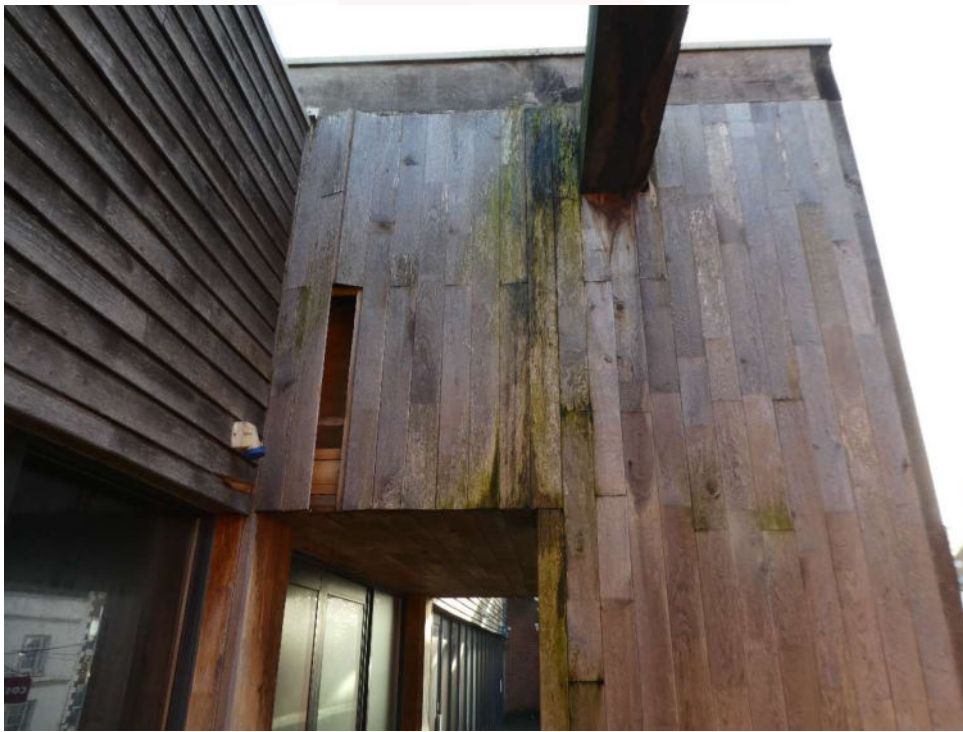
Photograph 2 – Timber façade arrangement to front of Civic Centre
