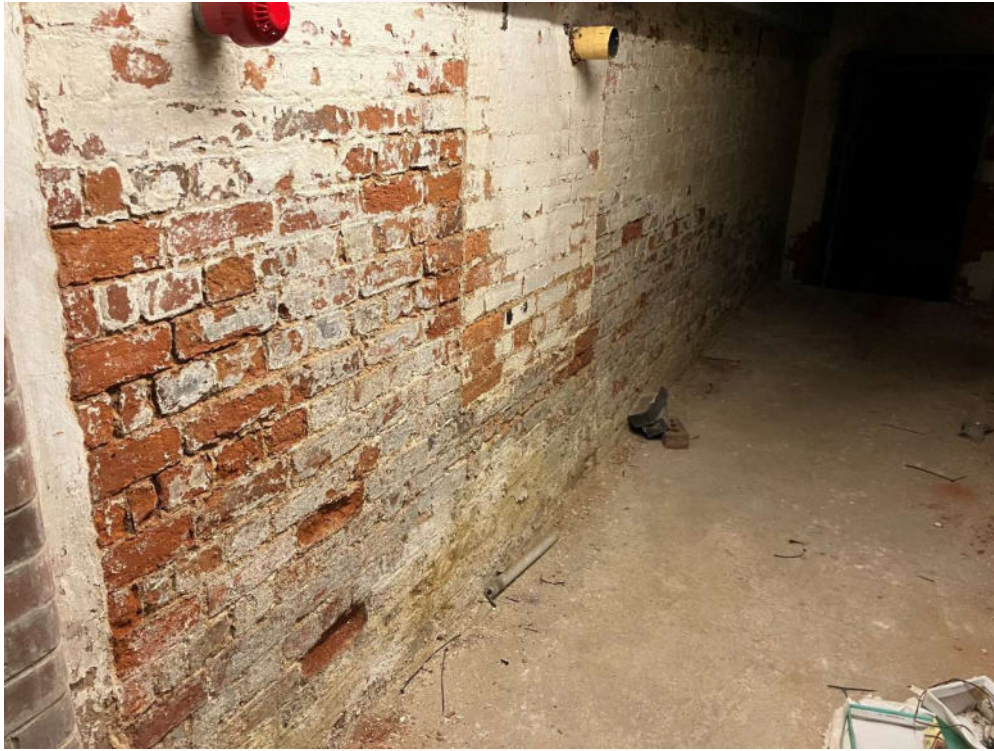
Photograph 31 – Typical condition of brickwork in basement – no change
