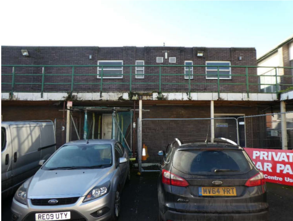
Photograph 4 – Rear elevation of Civic Centre with canopy present
