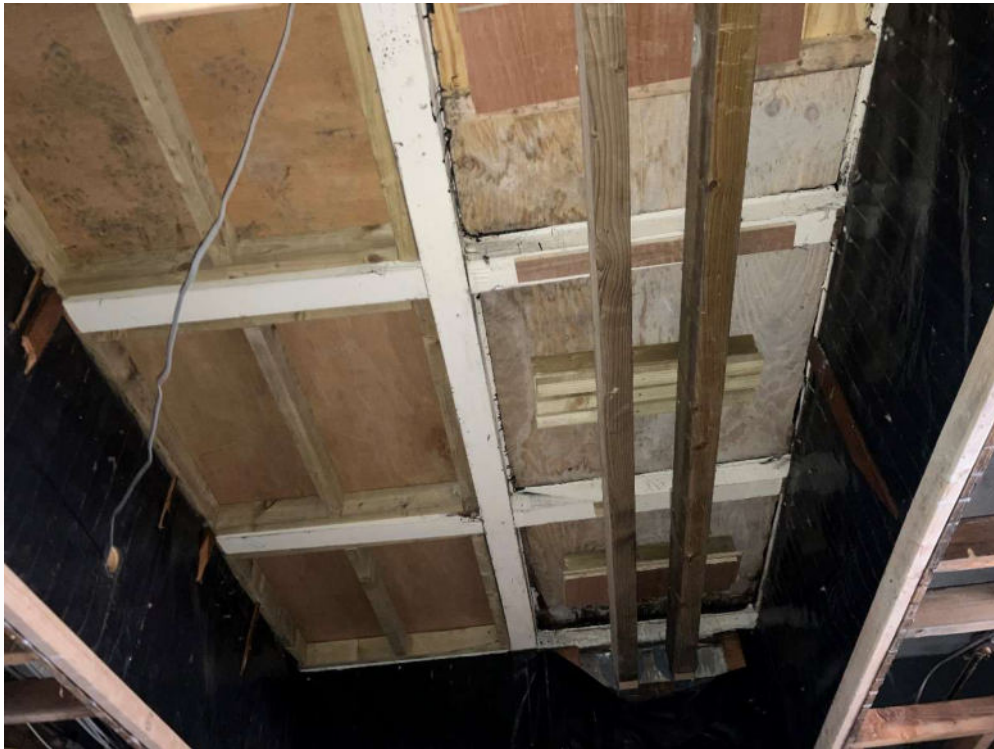
Photograph 47 – Section of timber roof to corridor by entrance to Civic Centre
