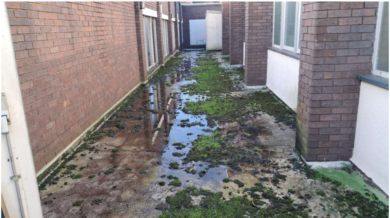
Photograph 15 – Right side elevation of Market Hall at high level above corridor (2026 update) – note standing water
