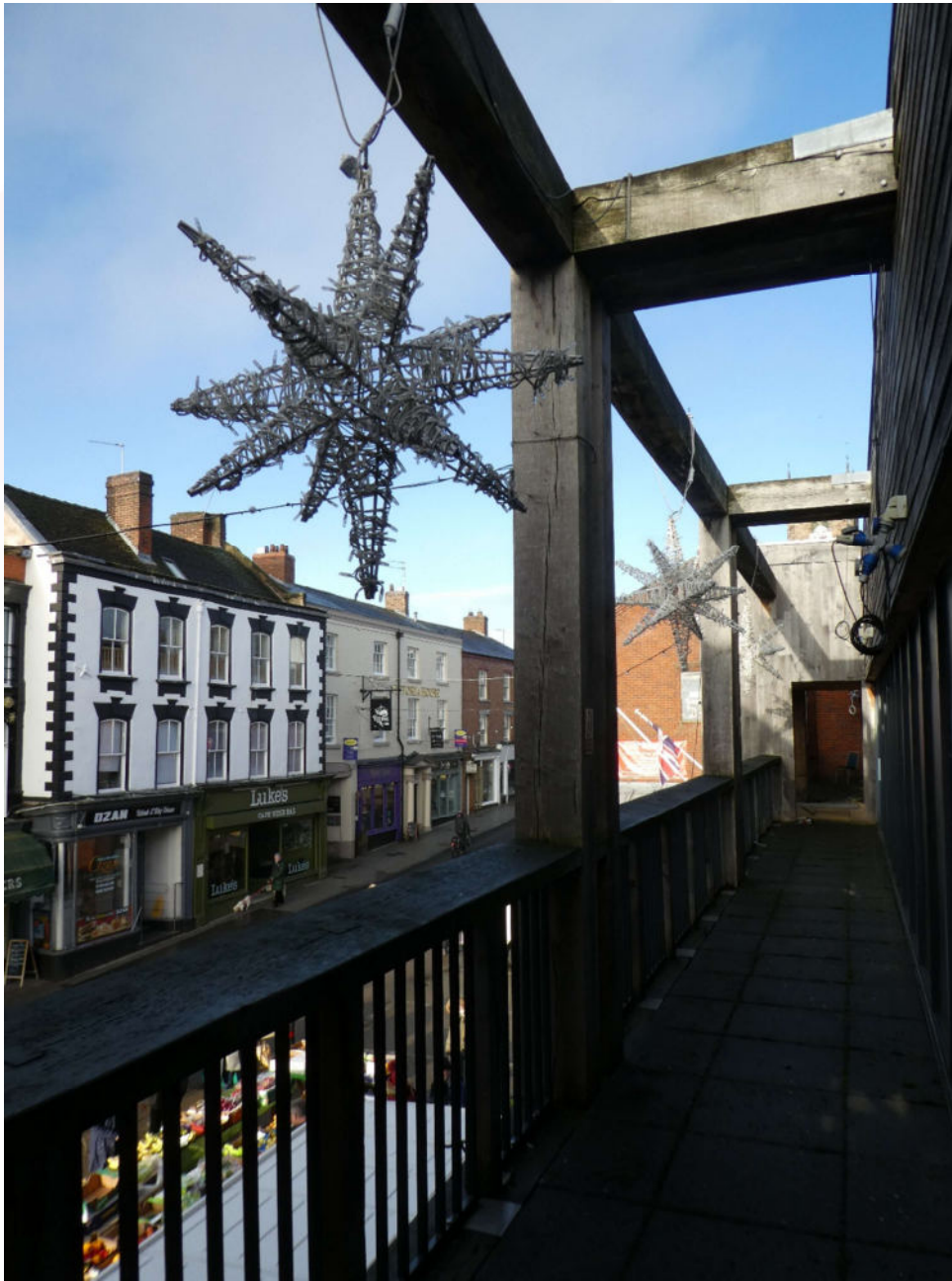
Photograph 3 – Balustrading arrangement to timber façade at front of Civic Centre
