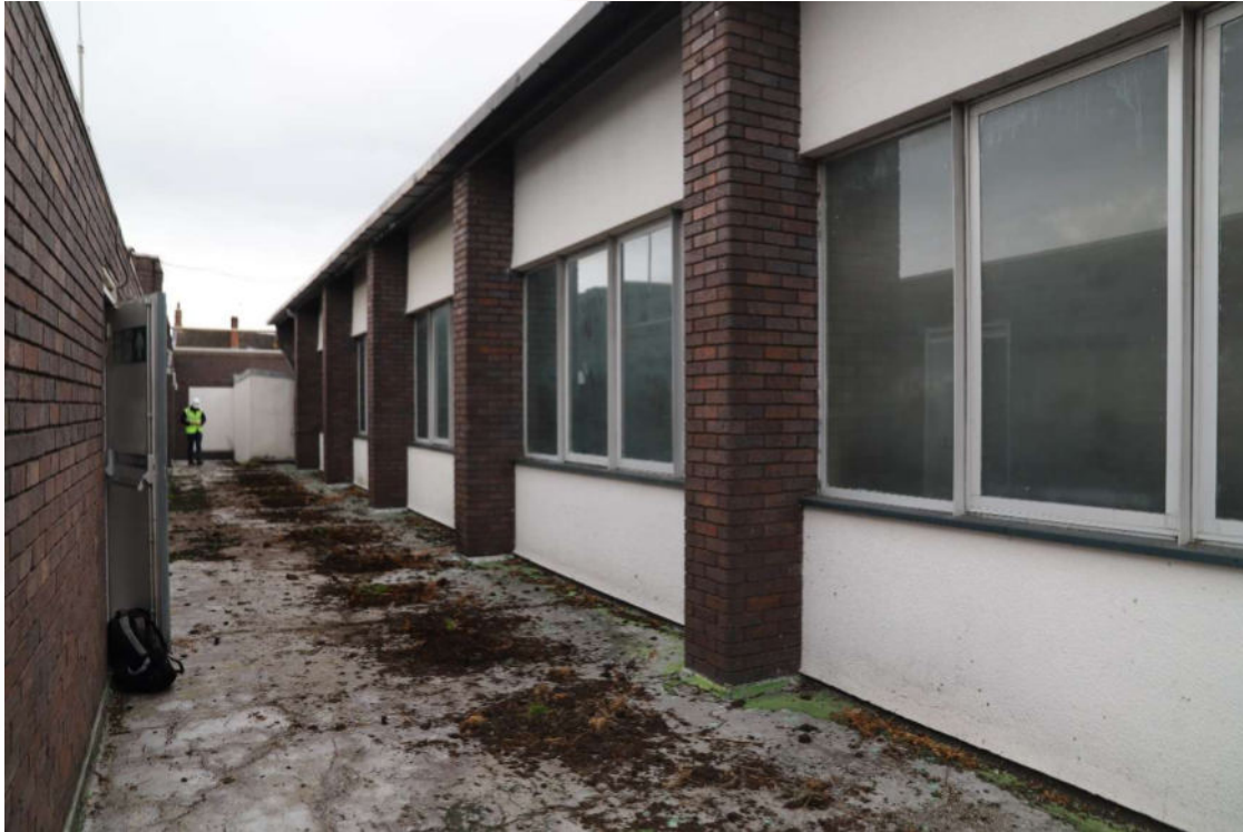
Photograph 14 – Right side elevation of Market Hall at high level above corridor (2024)
