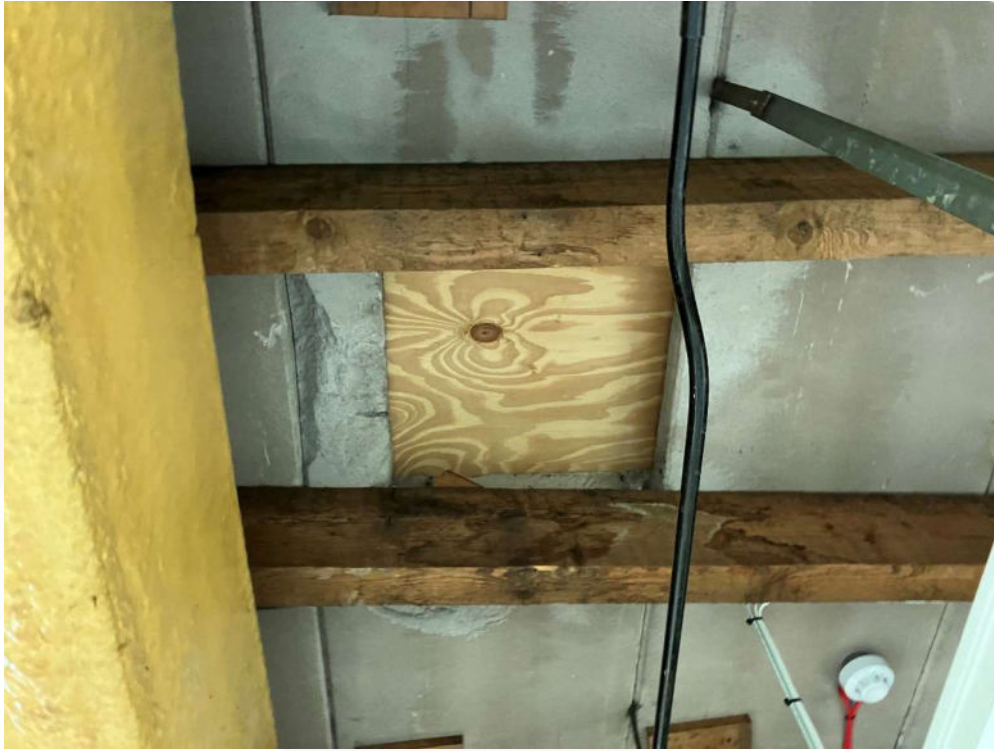
Photograph 37 – timber trimming to opening in roof over kitchen area to first floor – no change
