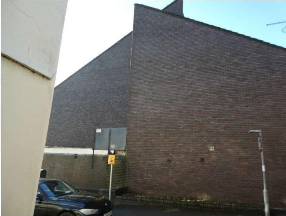
Photograph 10 – Rear elevation of Market Hall
