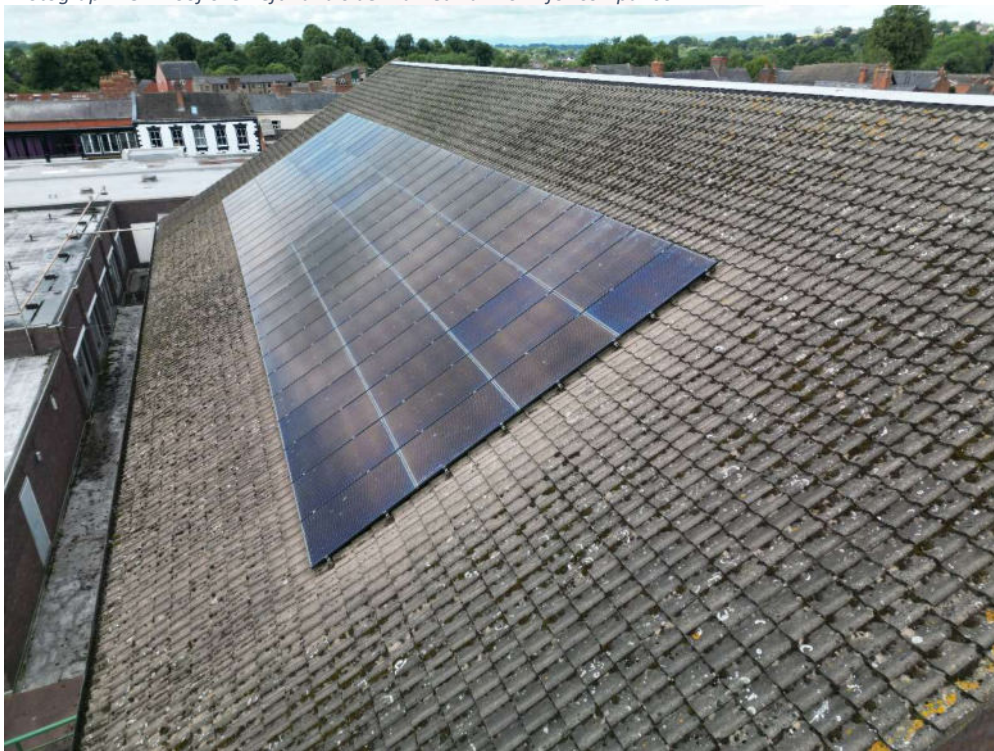
Photograph 29 – roof over right hand side Market Hall 2024 for comparison
