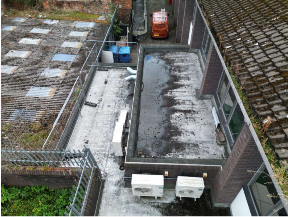
Photograph 26 – Roof over garage 2024 for comparison
