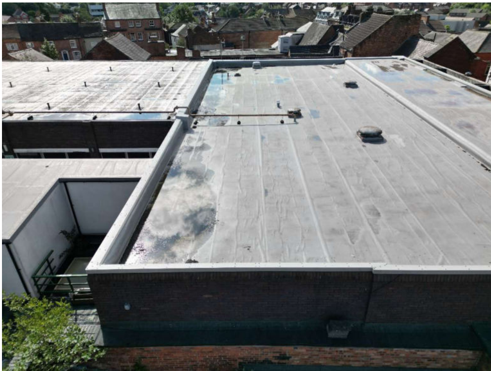
Photograph 23 – Roof over rear of Civic Centre 2024 for comparison
