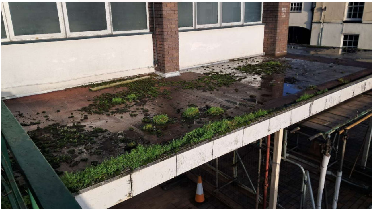
Photograph 13 – Top side roof of market hall walkway
