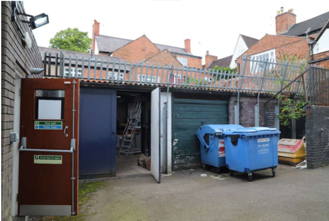
Photograph 20 – External Stores – no change
