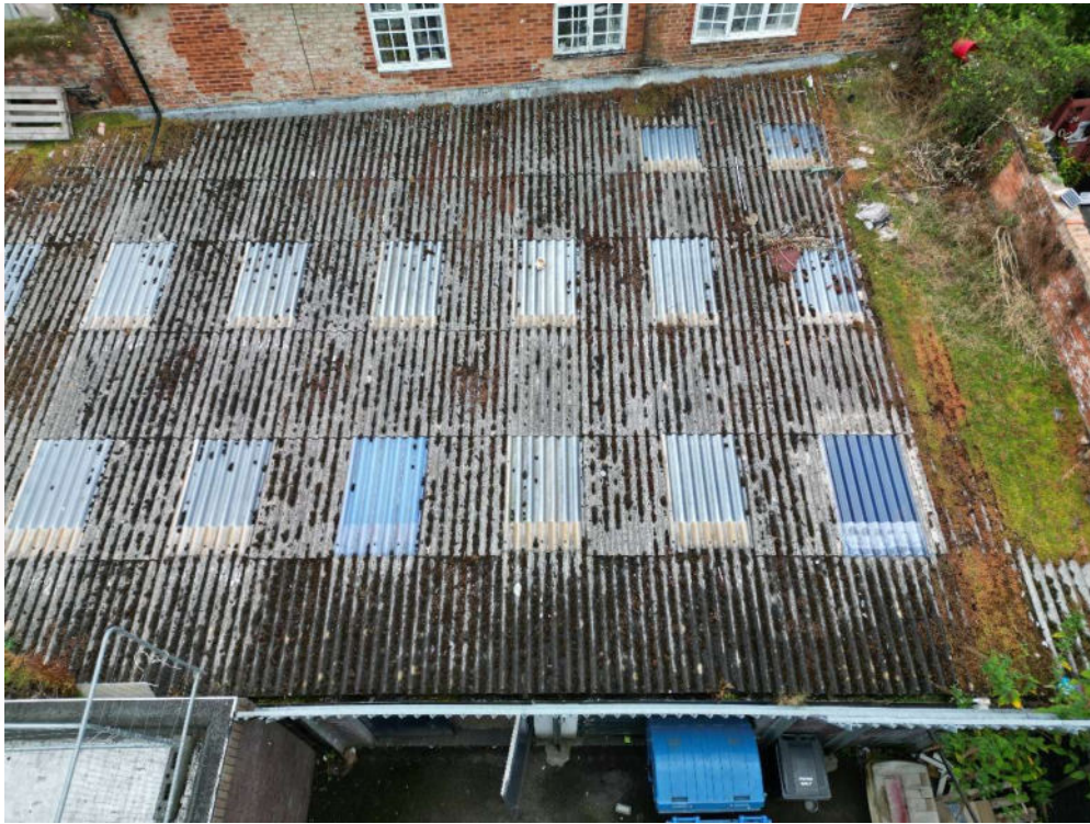
Photograph 30 – Roof over stores 2024 for comparison
