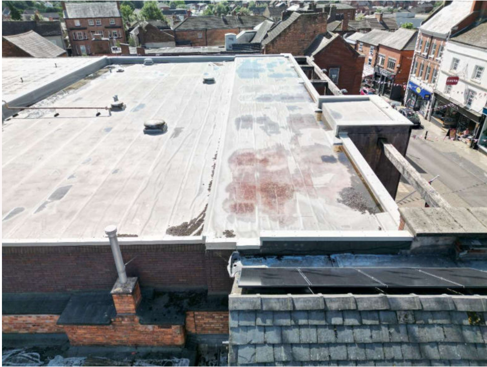
Photograph 22 – Roof over front of Civic Centre 2024 for comparison
