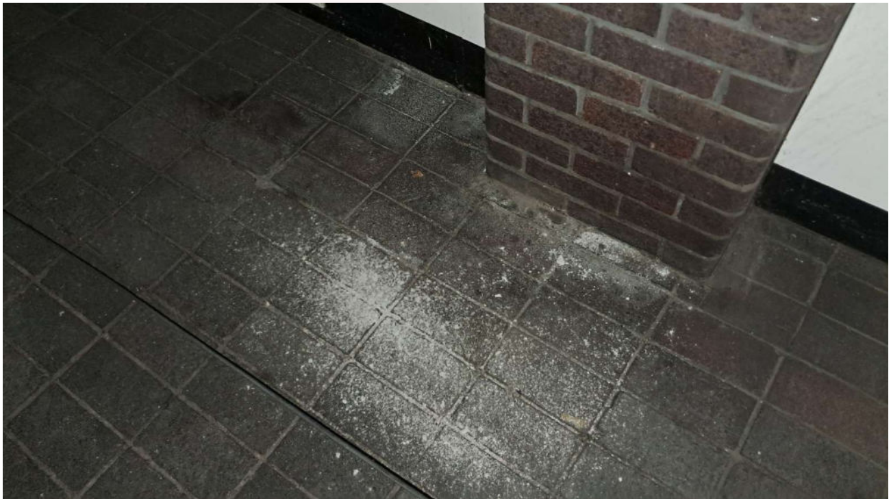
Photograph 46 – detritus on floor beneath trimming
